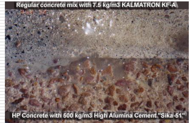
Regular concrete mix with 7.5 kg/m 3 KALMATRON KF-A HP Concrete with 500 kg/m 3 High Alumina Cement "Sika-51" Concrete floor of sulfuric acid dripping area after 9 months. Shown comparative application of concrete with 7.5 Kg/m 3 of KALMATRON® KF-A and concrete with 500 Kg/m 3 of High Alumina Cement R51, Lafarge.
