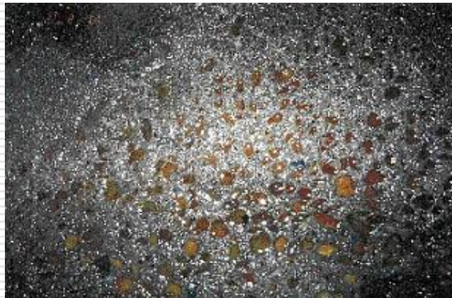
"Korvest Engineering" LTD Galvanizing Plant, AU "Cement matrix with KALMATRON® KF-A has been stronger than coarse aggregate." Repair of concrete floor damaged by hydrochloric acid and ammonium chloride solution by coating with concrete containing KALMATRON® KF-A
