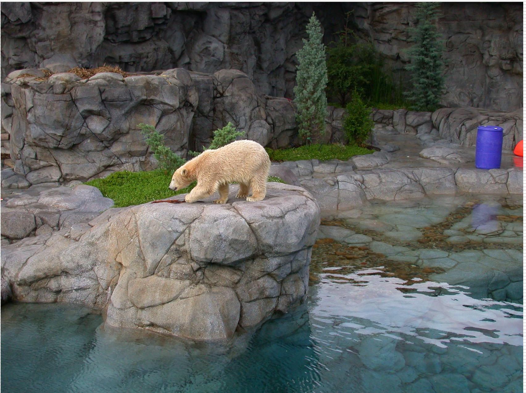
Polar Bear Shores. Sea World, Gold Cost, Australia. Completed – December 2000 Construction company – Streetscapes. Application: 30 MPa concrete mix with 7.5 Kg/m 3 of KALMATRON®KF-A, W/C=0.41 Description – artificial rock enclosure for polar bears in cooled sea-water. Result: after four years no signs of concrete degeneration. Typically degeneration begins to show after the first year.
