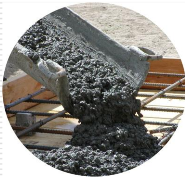
Conventional concrete flow
